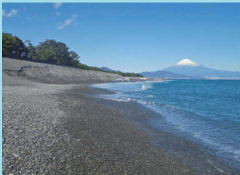
Erosion countermeasures at Miho no Matsubara
