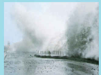
Wave overtopping a road during a typhoon
