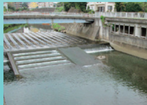
Forebay gate for the diversion channel of the Katabira River
